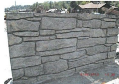
Concrete Form Liner Wall
