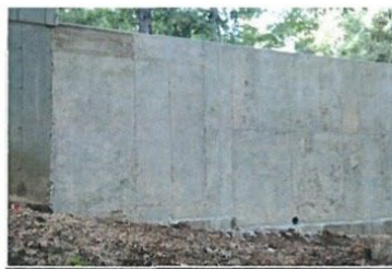
Smooth Concrete Wall
