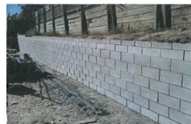
Smooth Face CMU Wall
